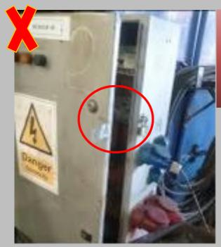
An original lock was broken in electrical distribution board
