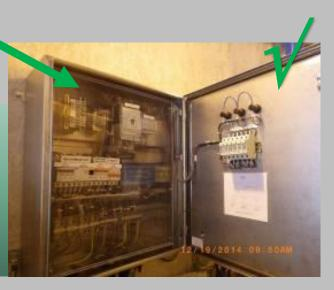
Electrical distribution board (DB) is installed with insulation board and ELCB/ RCCB
