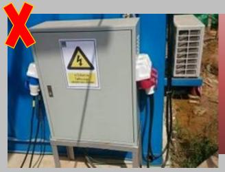
Without display electrician's name and contact on electrical distribution board (DB)
