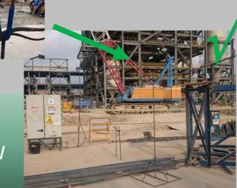
Electrical cable shall be hanged with insulated hooks
