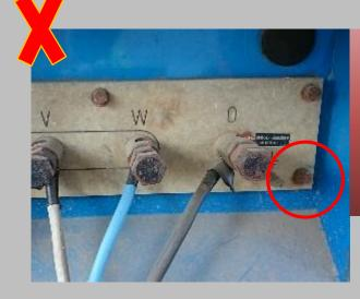
It is dangerous to use a generator without proper earthing
